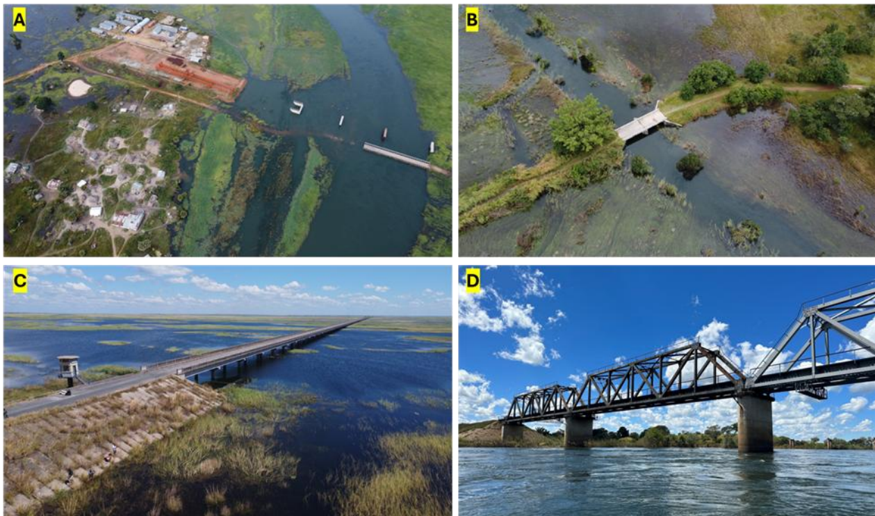
Figure 25. Bridges along the Chambeshi River transect: A) The Fwama bridge under construction; B) a small bridge in the upper reaches of the river; C) Tuta bridge, in the lower Bangweulu Swamps; and D) one of the three M1 highway bridges on the lower Chambeshi River.
