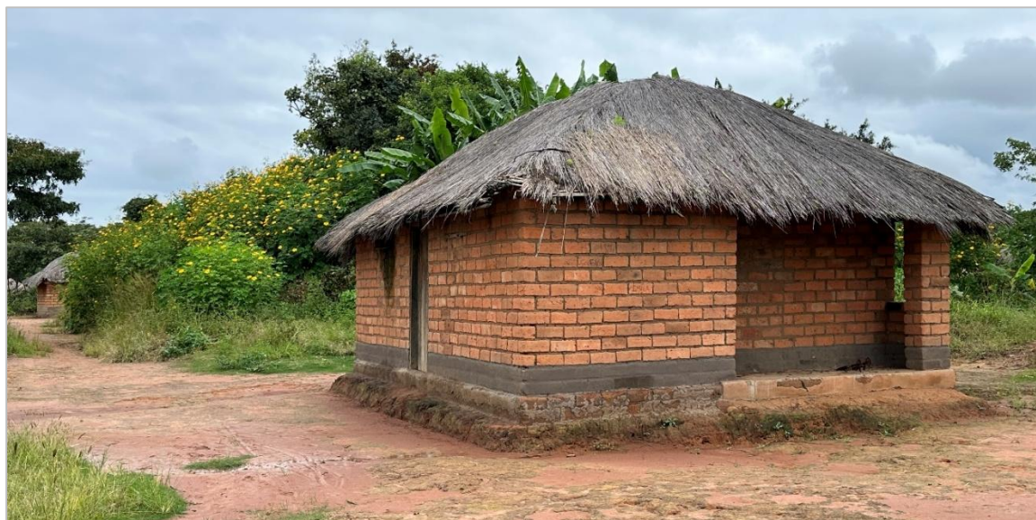
Figure 57. A typical building along the Chambeshi River.
