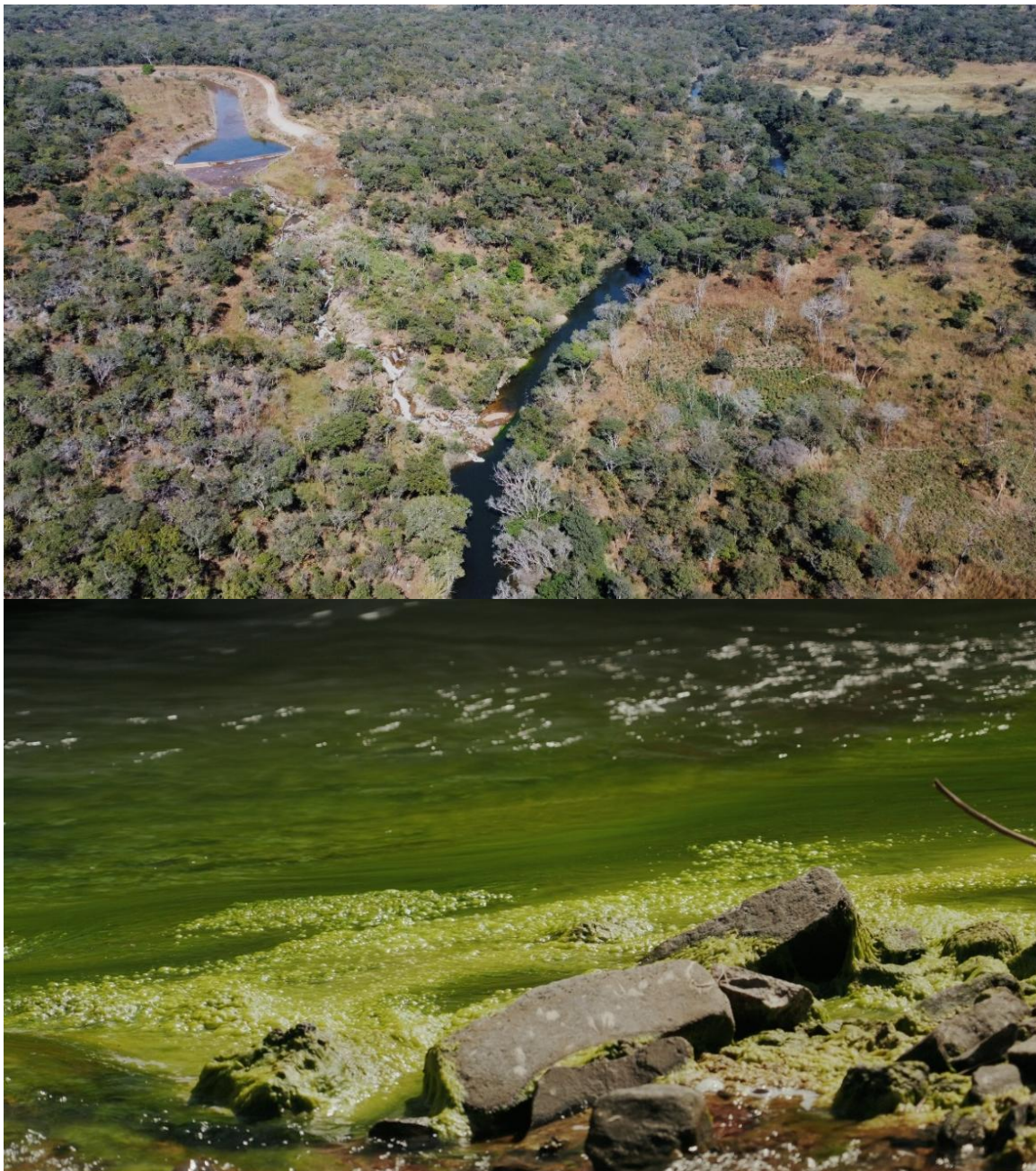
Figure 12. The Chisola mine tailings dam discharges directly into the Kabompo River, where bright green algae lined the banks.
