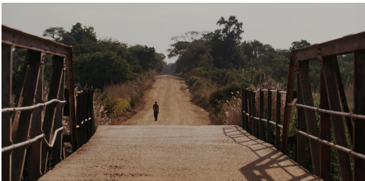
Figure 7. Kabompo River bridge near the settlement of Ntambu.
