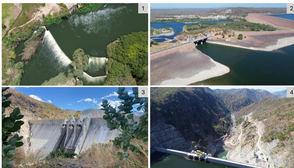
Figure 5. Some of the river infrastructure along the Kafue River. 1) a weir in the upper section of the river; 2) Itezhi-tezhi Dam and hydropower station; 3) and 4) Kafue Gorge Lower Dam and hydropower station.
