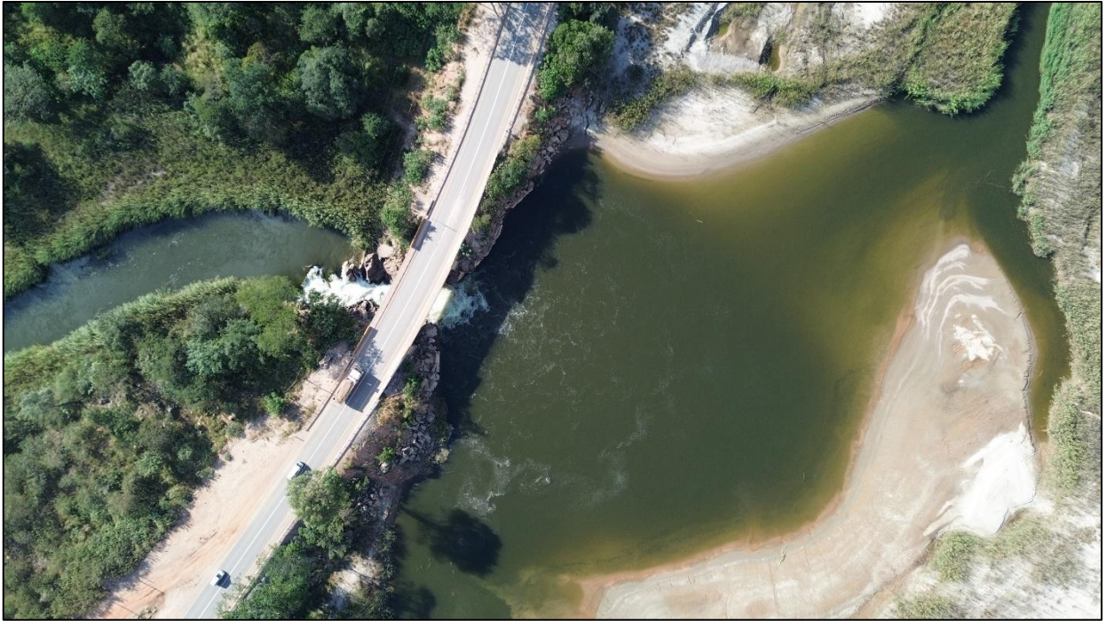
Figure 21. A motor vehicle bridge crossing the Kafue River.
